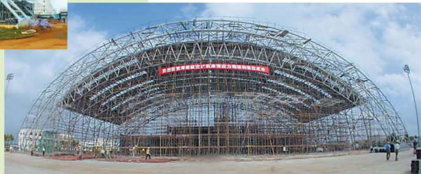
Maintenance Hangar#1 for Hainan Meilan Airport, China. (98-metre span stressed arch)
