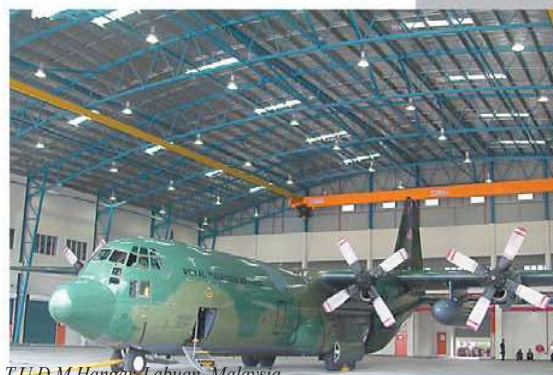
T.U.D.M Hangar, Labuan, Malaysia 4 nos 54m span stressed arch frame
