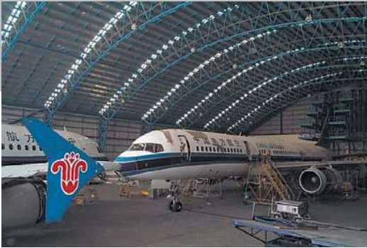
Gameco Hangar, Guangzhou, China (60-metre span stressed arch)
