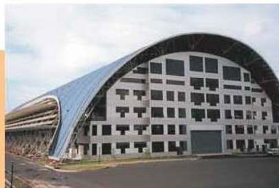
The Tenaga Nasional Research & Development Centre, Bangi, Selangor, Malaysia (83.5-metre span stressed arch)
