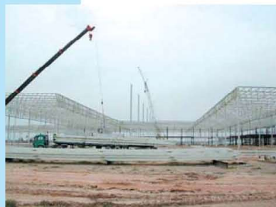
Naza Automotive Factory at Gurun, Kedah, Malaysia. • Engineer and erect in JV with Namfatt Fabricators Sdn. Bhd. • Steel tonnage : 3,000 tonnes
