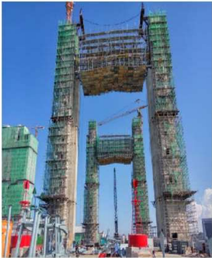
2nd Lifting for Structure at P4
