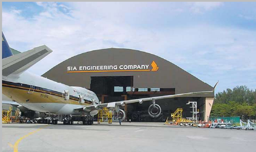
Single Bay Hangar for the SIAEC, Singapore (87-metre span stressed arch)
