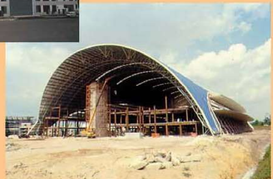
The Tenaga Nasional Research & Development Centre, Bangi, Selangor, Malaysia (83.5-metre span stressed arch)
