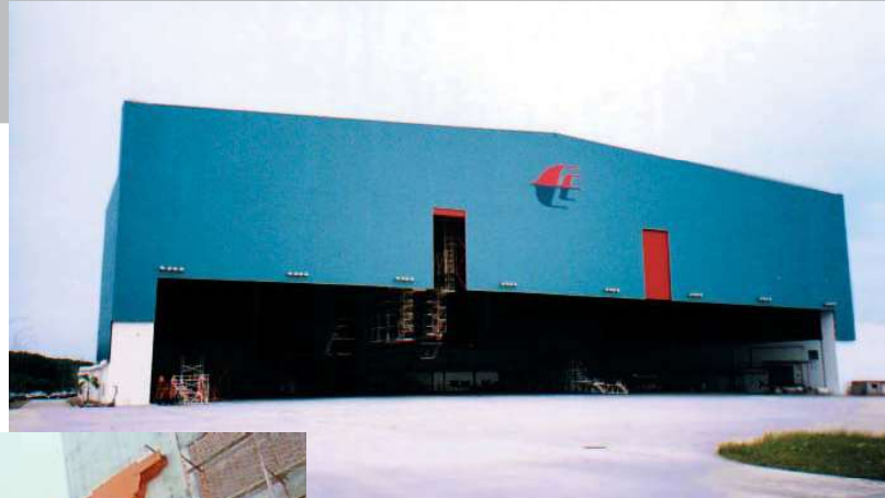
The Malaysia Airlines Hangar#4, Subang (2-bay 126-metre span)
