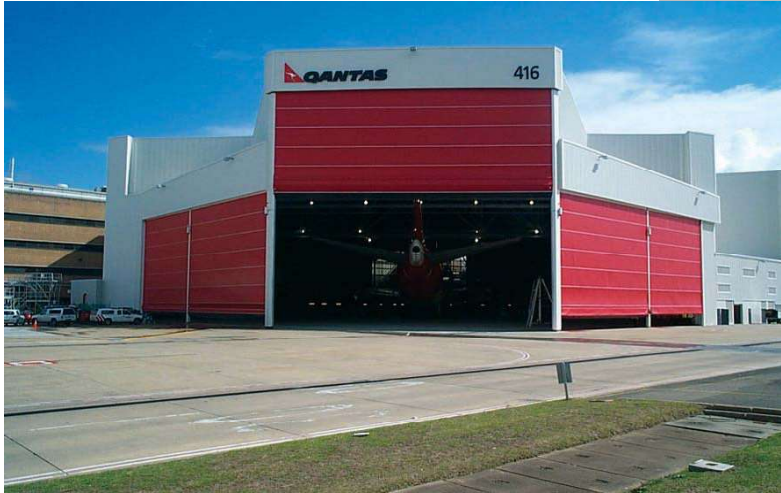
Mascot Hangar, Australia. • Engineering support for STRARCH International Limited • Steel tonnage : 758 tonnes
