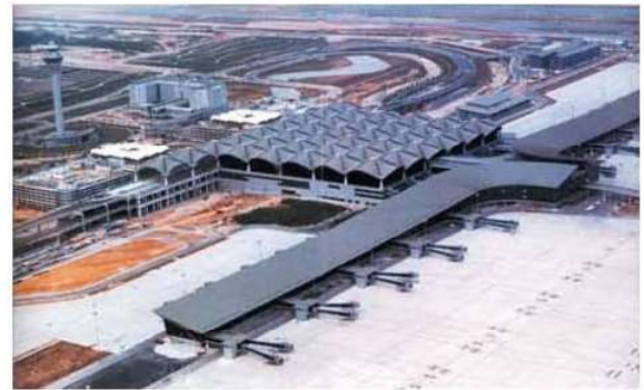
CP Building, Kuala Lumpur International Airport (Hall B roof structure)
