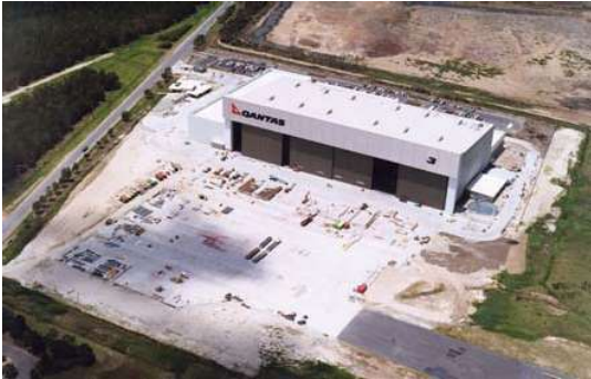
Qantas Hangar at Brisbane, Australia. • Engineering support for STRARCH International Limited. • Steel tonnage: 3,000 tonnes • 170-metre span 2 1 / 2 -bay Aircraft Hangar
