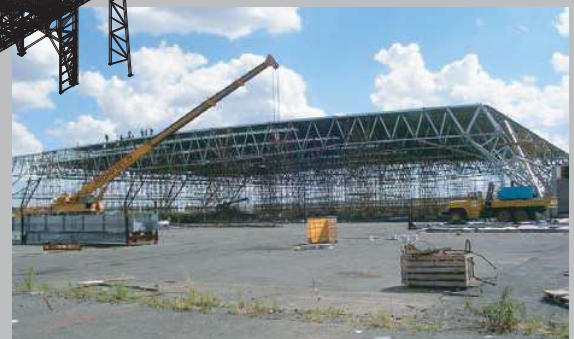
Kenya Hangar at Nairobi, Kenya. • 80-metre x 80-metre span stressed arch
