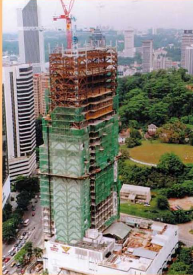
The Weld, Kuala Lumpur (25-Storey steel-framed building)
