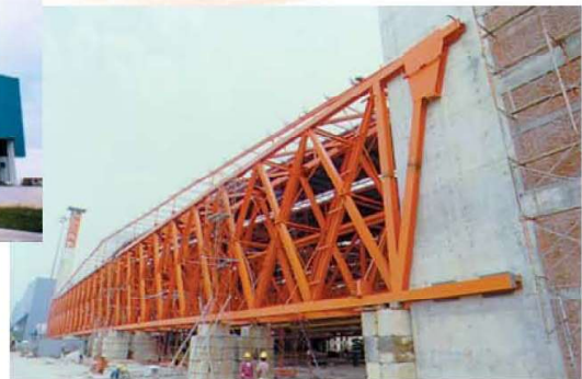
The Malaysia Airlines Hangar#4, Subang (2-bay 126-metre span)
