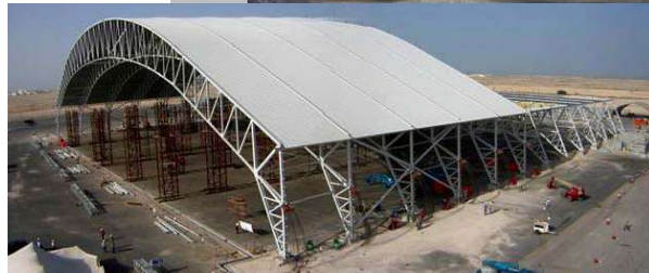
Amiri Flight - Qatar Airways (155-metre clear span x 140-metre deep)
