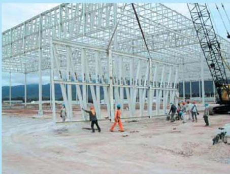
Naza Automotive Factory at Gurun, Kedah, Malaysia. • Engineer and erect in JV with Namfatt Fabricators Sdn. Bhd. • Steel tonnage : 3,000 tonnes
