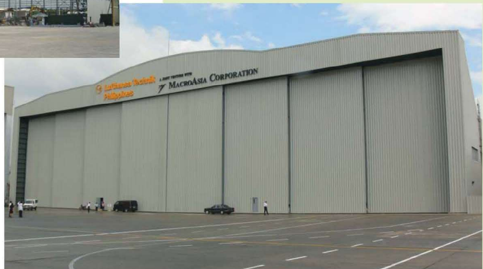
One Bay Wide Body Aircraft Hangar Lufthansa Technik Philippines Villamor Air Base, Pasay City, Philippines.
