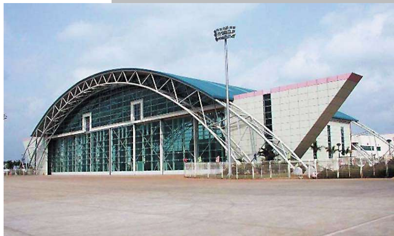
Maintenance Hangar#1 for Hainan Meilan Airport, China. (98-metre span stressed arch)
