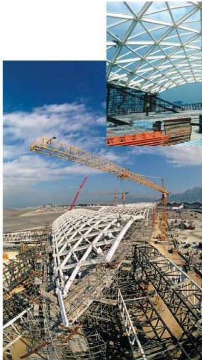
Hong Kong International Airport (Northwest concourse roof structure)
