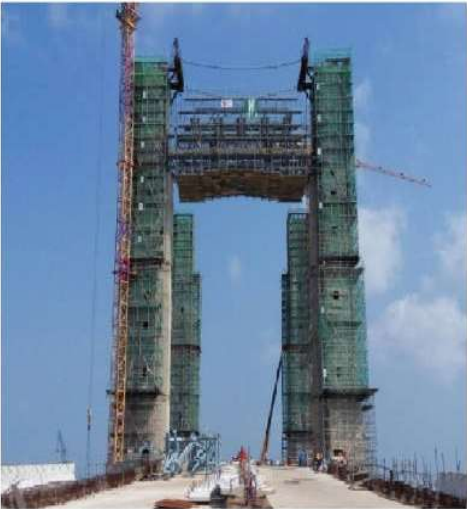
1st Lifting for Structure at P5
